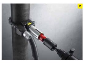
2. Drill the hole with the drilling machine and remove drill guide.
