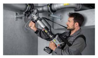
Enables pressing of thick-walled steel up to 4 inch: the Pressgun Press Booster.
