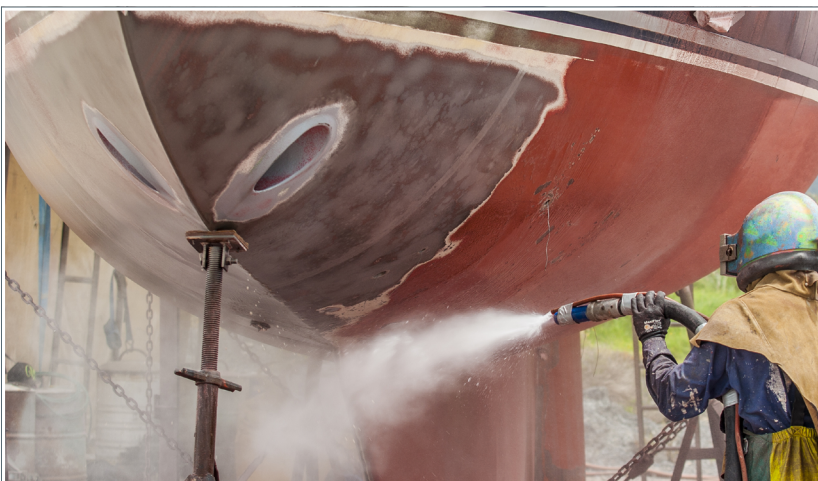
Fig. 119: Active air for sandblasting
