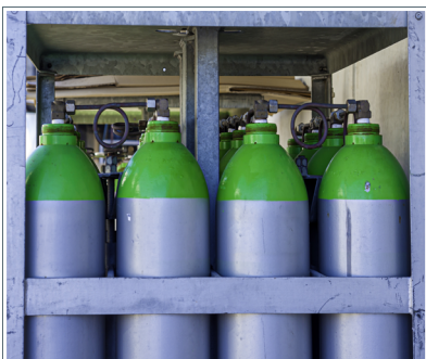
Fig. 147: Secured liquid gas cylinders
