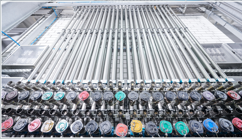
Fig. 173: High number of cooling lubricants managed using Viega Sanpress Inox G
