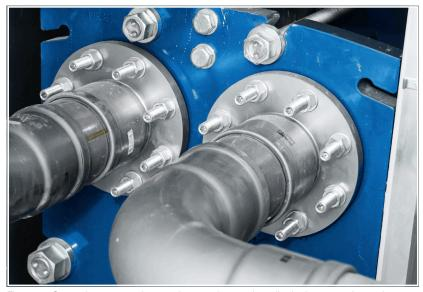
Fig. 103: Secondary connection to a heat exchanger in a district heat transfer station
