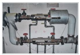
Fig. 81: Filter system (redundant design)
