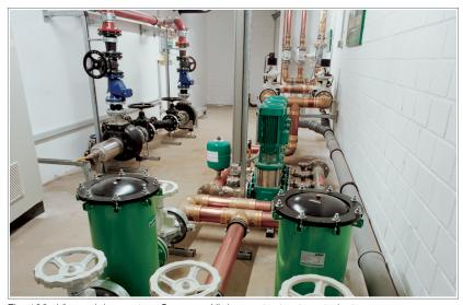
Fig. 100: Viega piping system Sanpress XL in a water treatment plant
