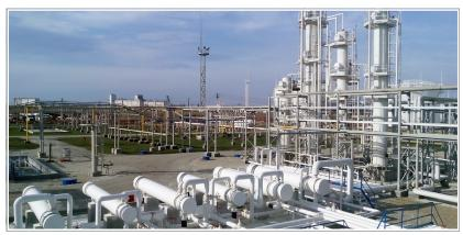
Fig. 160: Distillation column in a crude oil refinery
