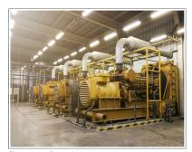
Fig. 170: Diesel-operated emergency generator
