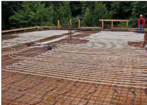
Fig. 212: Fonterra Active, construction site photo
