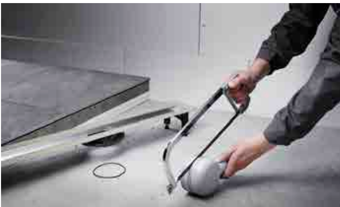
The standard drain can be converted on site into a reconstruction model by simple cutting it to height.
