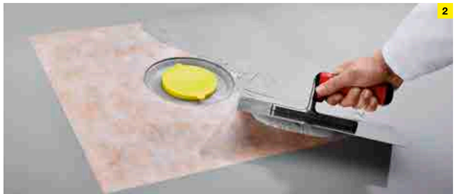
Application of the 2 nd sealing layer with a two-component plastic cement mortar combination proven in building practice.
