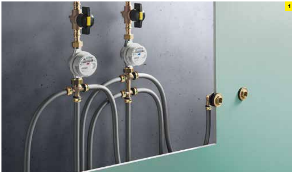
Raxofix wall lead-ins for drywall installation and pre-fabrication of bathroom units.
