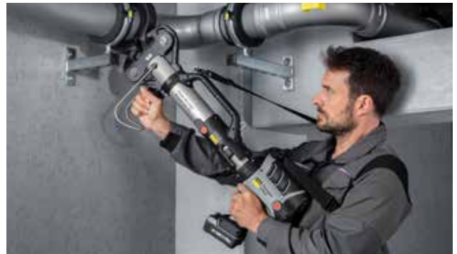
Enables pressing of thick-walled steel up to 4 inch: the Pressgun Press Booster.
