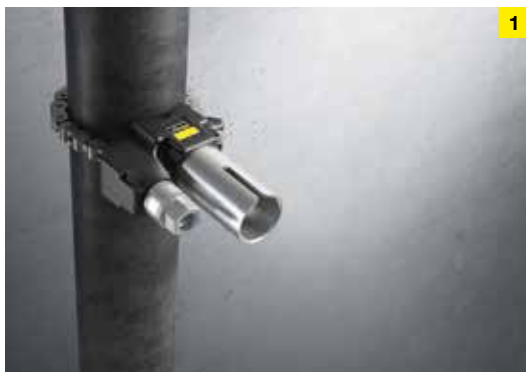
1. Attach a special drill guide on the steel pipe to guide the drilling shaft.
